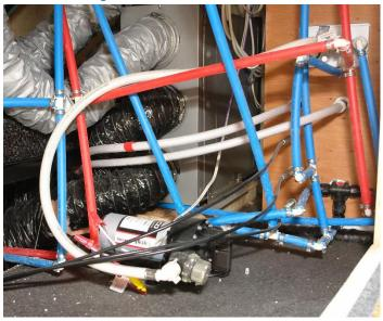
The water pump is located on the floor behind the UDC. When winterizing, the pump will suck antifreeze in and pump it through the water system (but not into the fresh tank or through the black tank flush systems). However, if using compressed air to winterize, you must take additional steps to protect the water pump and its filter assembly. Consult our <u>Winterization Guide</u> for details.
