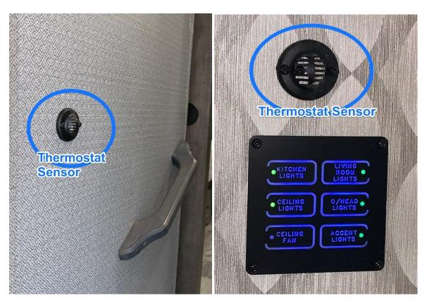
While you may have three thermostats, with each thermostat controlling a separate air conditioning unit, only one of those thermostats is used with the furnace controls. Unlike older models with separate thermostats, the KIB Touchscreen or phone app will manage this for you.
