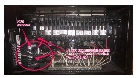
If it detects a voltage differential across L1 and L2, it interprets that as 50 amp service. If it does not detect a voltage differential, the system will assume that both legs are being supplied by a single source. In that case, the system defaults to a 30 amp setting. If plugged into a 20 amp circuit, you must set the controller to 20 amps manually. If you don't set it to 20 amps, the controller will operate as though the power source was 30 amps and you may experience power issues.
