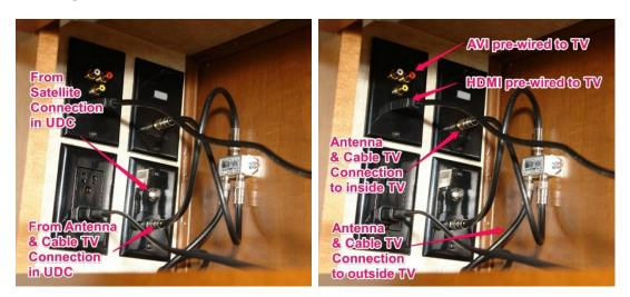
The satellite COAX connection would be wired to the input of your satellite receiver. The output of the satellite receiver would go to one of the open connectors on the wall plate. Newer receivers would probably use an HDMI output to the HDMI connector on the wall plate as shown above. Note that on
