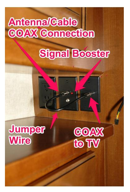
The signal booster amplifies the weak signals from the antenna and must be ON in order to receive over-the-air signals. However, when using cable TV, the signal booster must be OFF. It's important to set the signal booster correctly before attempting a channel scan on the TV.
