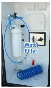
Landmark 365 units come with a single-stage water filter located inside the Universal Docking Center (UDC).
