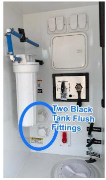
The black tank flush allows you to run campground water through a sprayer mounted inside the black tank(s) in order to help clean out the tank.
